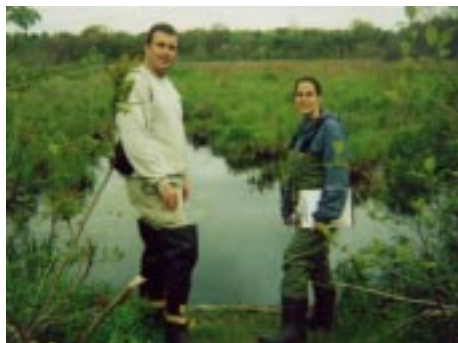
Rick Dawe of the Lynn Water and Sewer Commission and SRWC Director Joan LeBlanc inspect culverts in Reedy Meadow, June 2005.
